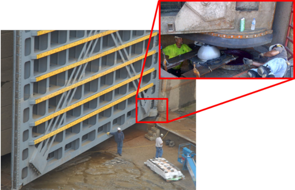
Figure 3. Pintle of a Miter Gate [14]
