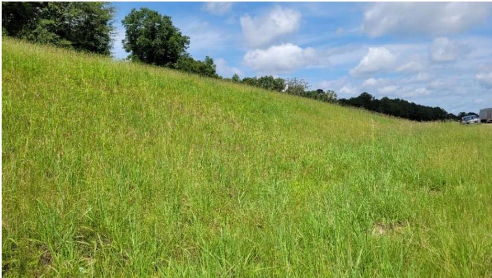
**Figure 2.7** Vetiver stabilizing a previously failed highway slope in Mississippi.
