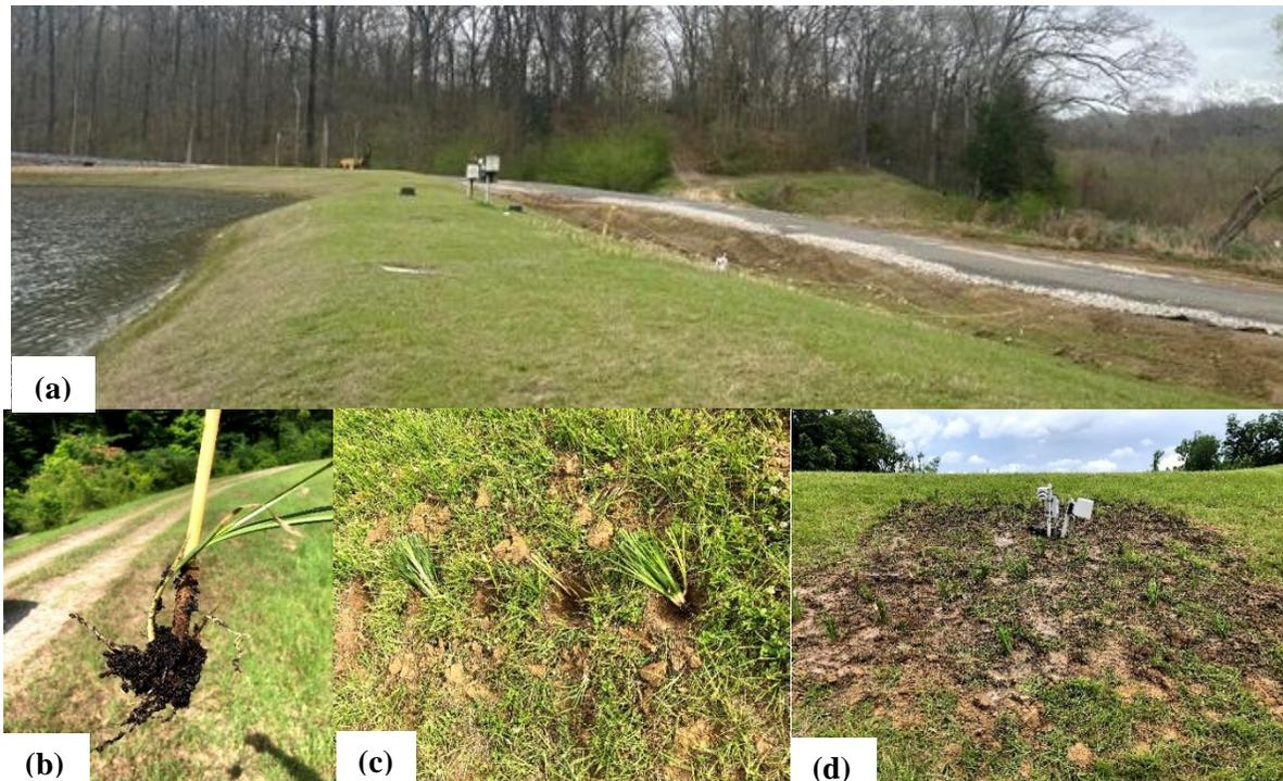
**Figure 4.2** Planting vetiver on test levee at ERDC: (a) looking east, (b) vetiver tiller before planting, (c) planted vetiver, and (d) looking north after planting
