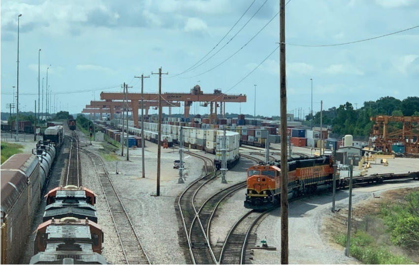
Figure 6: The BNSF Railway Intermodal Facility in Memphis, TN.
