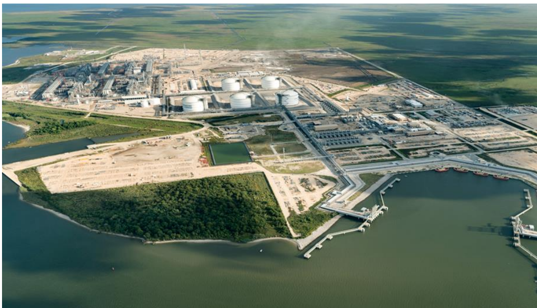
Figure 5. Cheniere's LNG Export Terminal, Sabine Pass, Cameron Parish, LA. Source: Cheniere Energy 2016.
